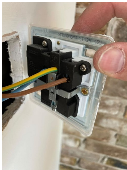
Inspecting a socket-outlet
