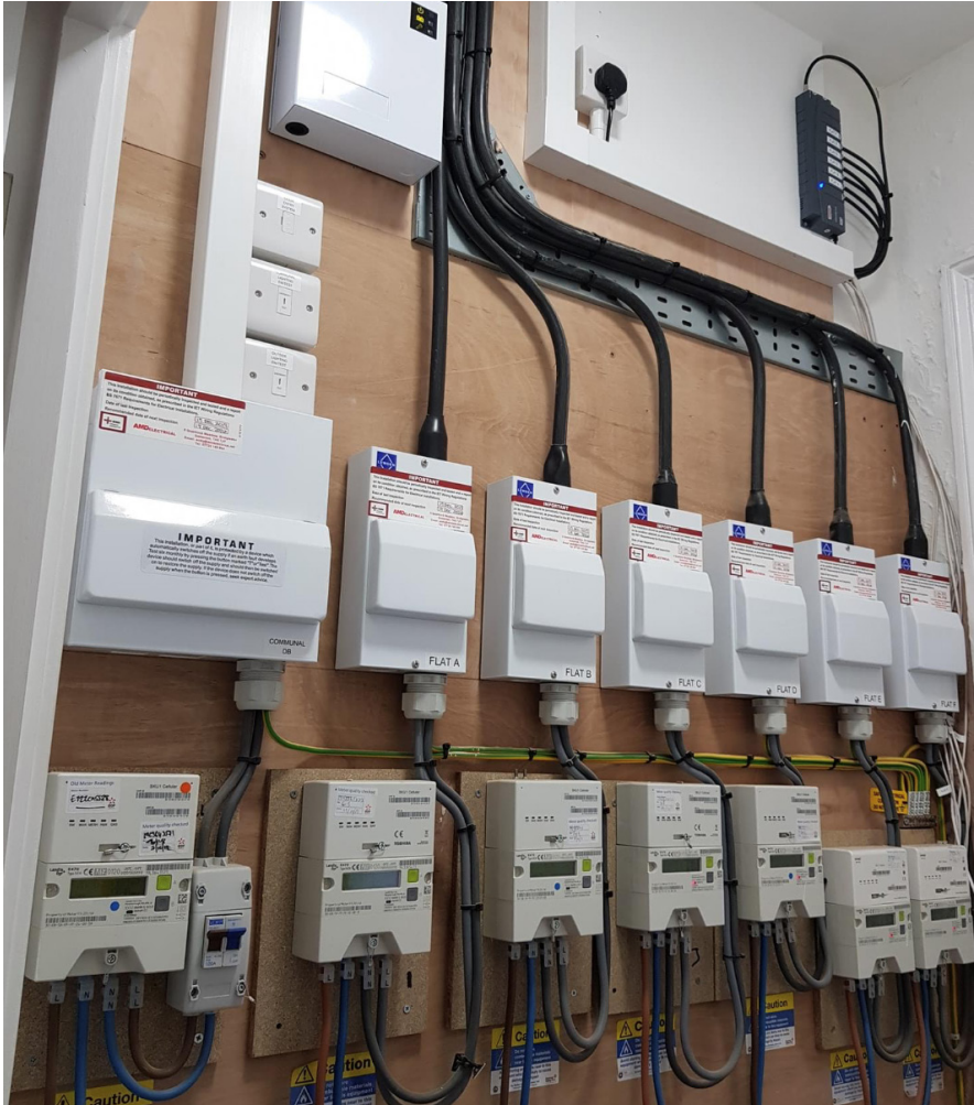
Figure A1: Example of group metering at the electrical intake position/origin. Photo courtesy of AMD Electrical
