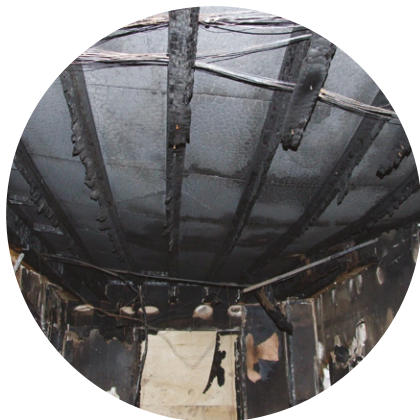
Result of an eight minute fire on lightweight joists (Courtesy of Manchester City Council - Building Control)
